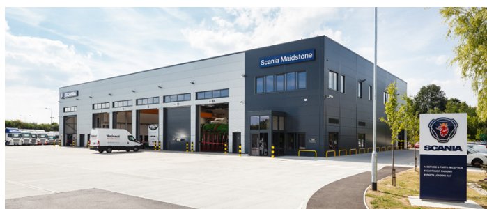
Scania Junction Six, Maidstone completed by GDM in 2016
